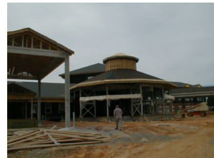
Building the Manor in 1999
